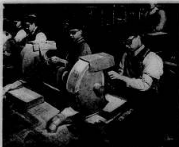
Hand Edging Smooths Away the Last Roughness
