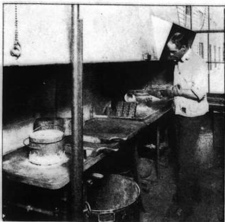
"White Magic." Pouring the Molten Gold into Molds
