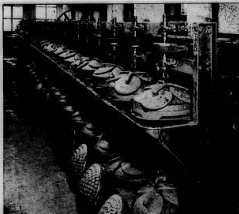
Machines of this kind Grind and Polish the Lenses
